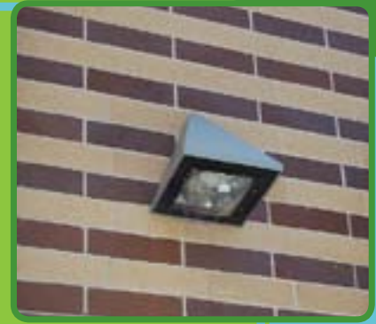
Above: Sloped light fixture deters birds from building nests.
