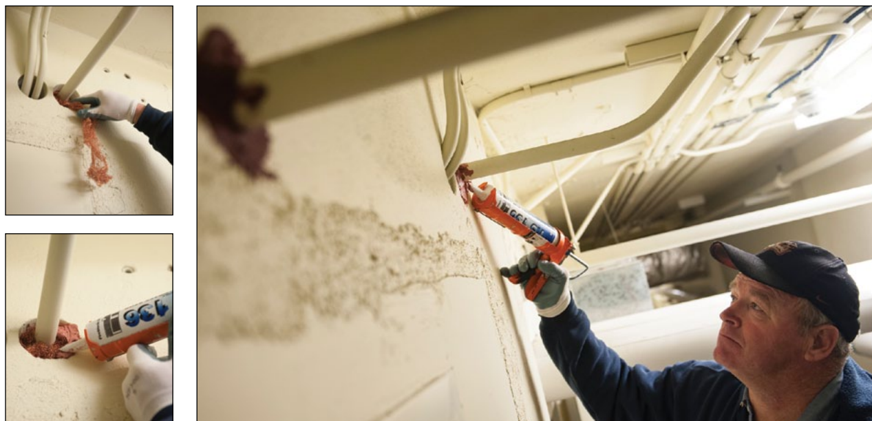
Figure 2. One way house mice find their way into a building is through gaps created for plumbing and wiring. Gaps of ¼ inch or more should be filled with Xcluder cloth or Stuf-fit copper mesh, then sealed with a silicone or polyurethane sealant.
