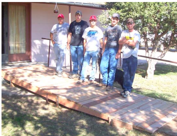
Springfield FFA showing off the new ramp they built and installed
