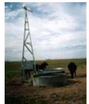
Turbine and Water Tank
