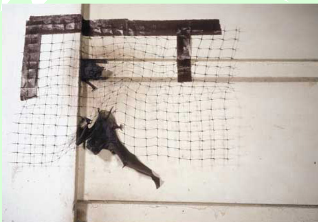
Bat exclusion with mesh (M. D. Tuttle, UC Statewide IPM Project)
