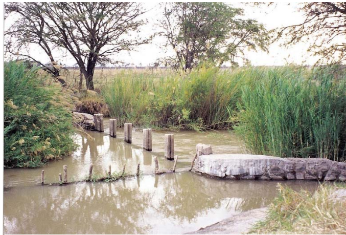
Fig. 38. A Farmer Built Diversion Structure to Divert Water To Their Unofficial Rice Irrigation Scheme
