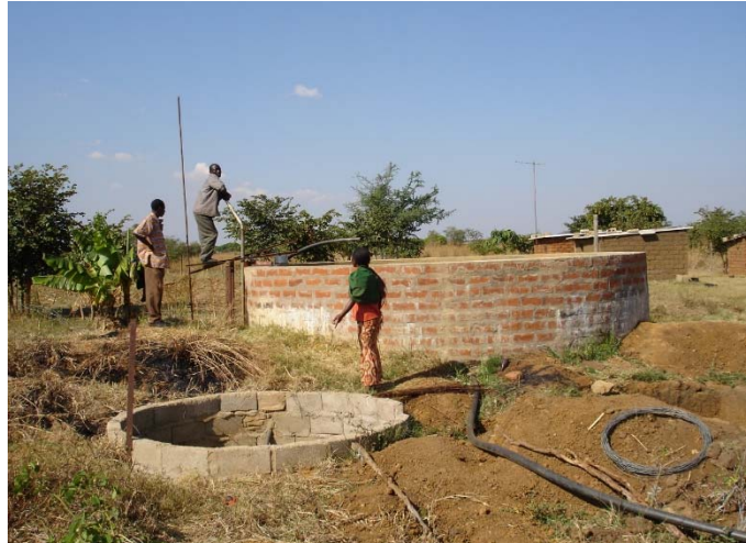
Fig. 34. Water Storage Built to Hold Irrigation Water for Use On Vegetables in Zambia. Note the Farmer Filled It With Small Diesel Pump Similar to that Used By Mr. Simon, and Not the Treadle Pump
