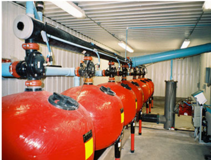
Fig. 4. Bank of sand filters for filtering water for commercial large scale drip system, even when using well water with limited suspended particulate material.
