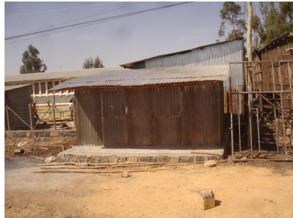
Fig. 23. Shop Being Prepared for Butter Sales, but Needing Improve Convection Circulation to Reduce Overheating.
