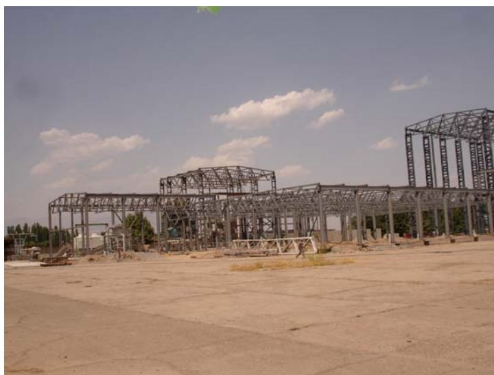
Fig. 1. Geha Foods Tomato Processing Facility under Construction
