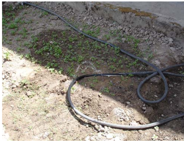
Fig. 20. Water spouting from a simple hole in a hose with no means for pressure compensation.
