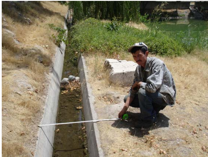
Fig. 17. Prefabricated canals commonly used in Tajikistan for moving surface water that have the potential to be used for gated head ditches by installing ports near the top of the section. The example is approximately 60 cm across the top as shown by the individual hand being at 1 m.
