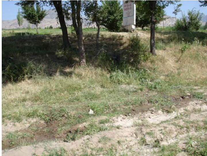
Fig. 12. Water coming from a cut into the canal down a bank to get to the very small head ditch.
