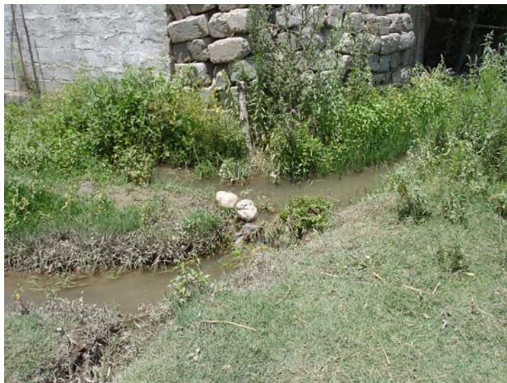
Fig. 11. A similar improvised control structure to divert water, but with considerable leaking occurring.
