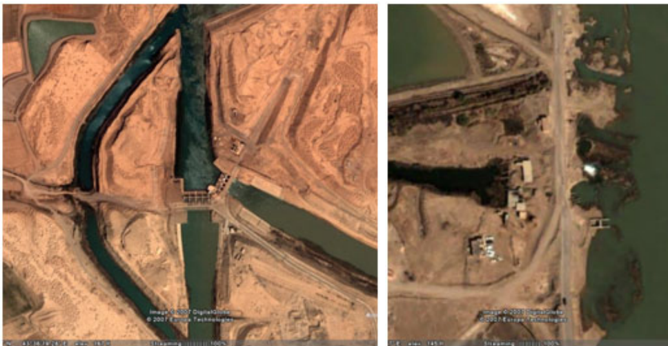
Fig. 2 & 3. The control structure in the main canal and pumping station lifting water into the secondary canal for the ICA.
