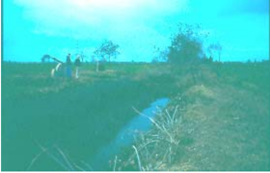
Fig. 26. Tertiary canal with weeds completely removed until the inlet for the sakia, but fully retained after the sakia inlet.
