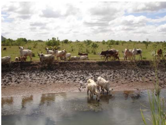
Fig. 20. Cattle drinking from the main canal and slumping the canal bank into the bottom reducing the canal conveyance capacity.
