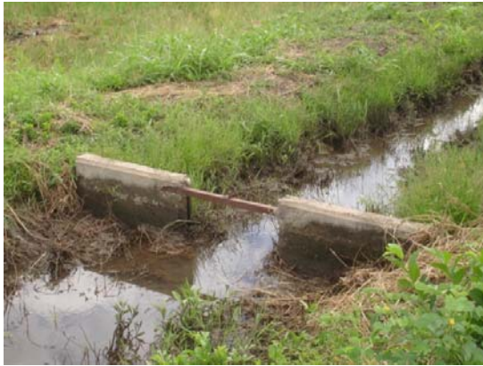
Fig 23 Concrete control structure for controlling water into tertiary canals.
