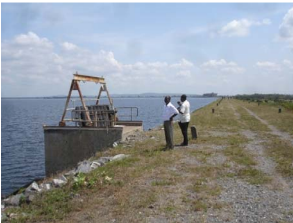
Fig 1. Inlet structure to the Irrigation scheme with the electric power plant in the distant background.
