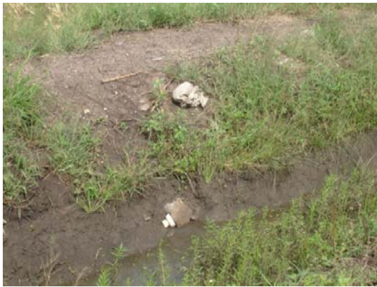
Fig. 27. Field inlet as simple pipe with plug for when water was not desired.
