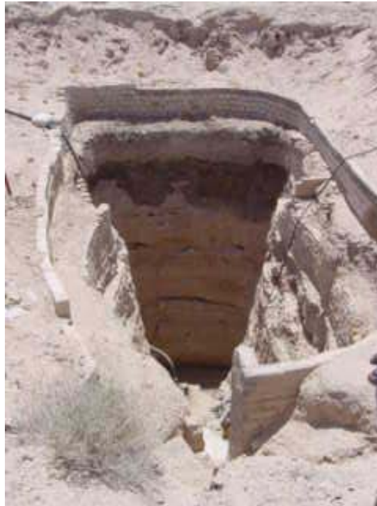
Fig. 12. Dug well in Basra, Iraq used for drip irrigation of tomatoes. Note pump at bottom of the well.
