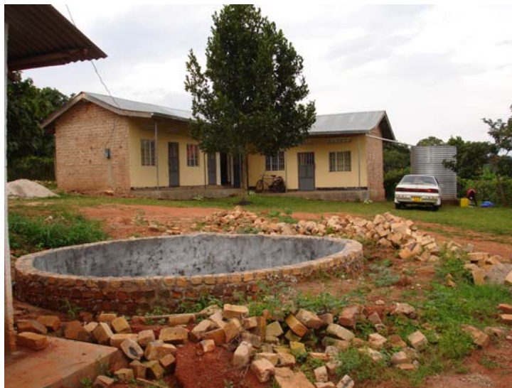
Fig. 20. Storage tanks at RUCID to collect rainwater from roof in background and below ground tank in foreground.
